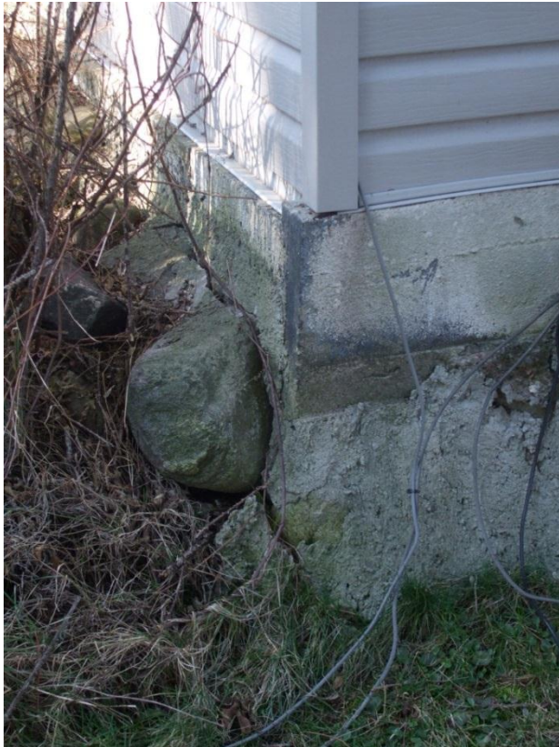
Photograph 16. Field stone foundation reinforced with concrete
