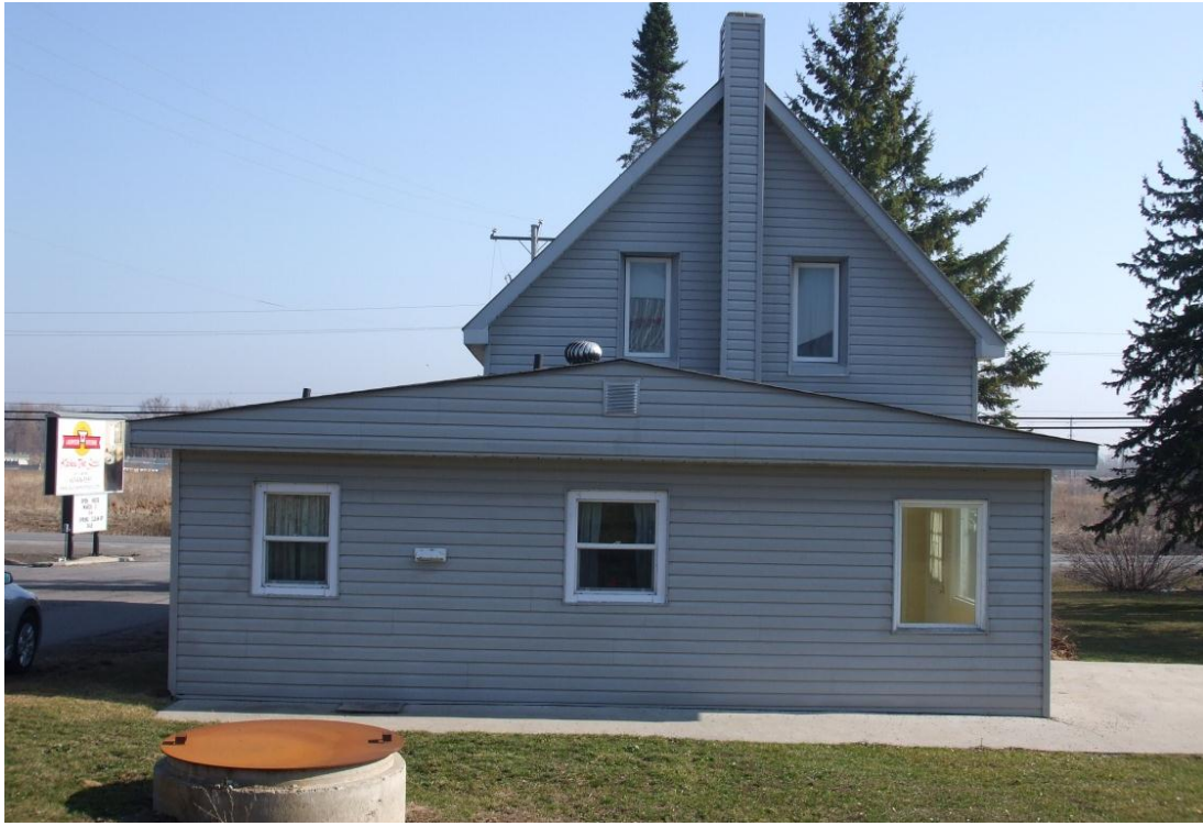
Photograph 14. Rear (west) elevation
