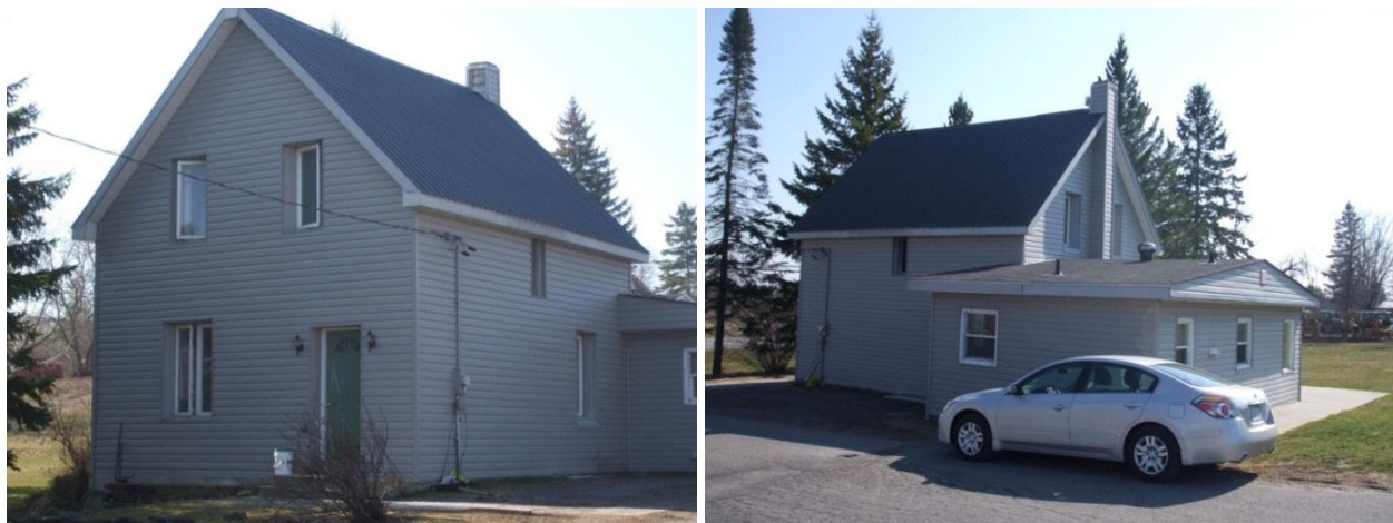
Photograph 11A and 11B. Showing the front and rear of the house.
